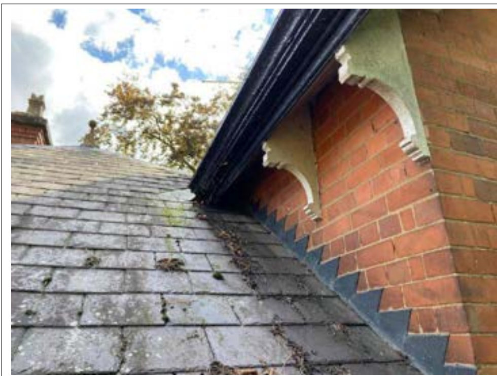
119. Decay to gutter lines.
