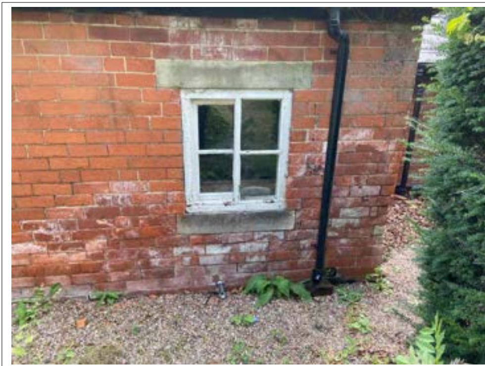
122. Rear of outhouse, efflorescence noted to brickwork.
