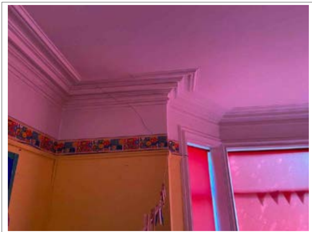
185. Cracking noted internally to front bay.
