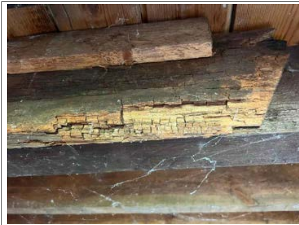
116. Decay noted to suspended ground floor timbers,
