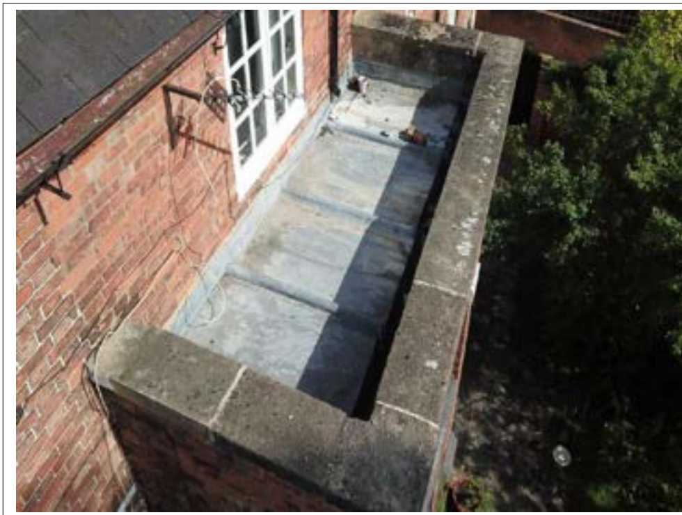
133. Leadwork to front parapet.
