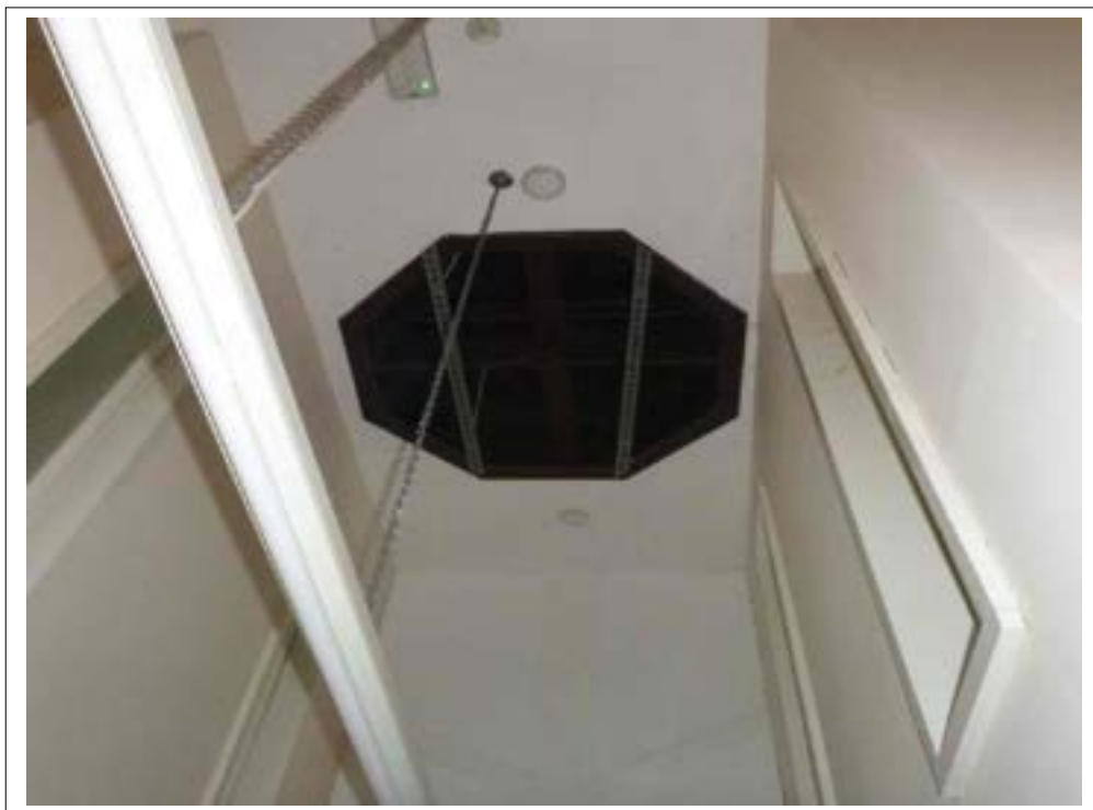
60. Support joists for roof cowels.
