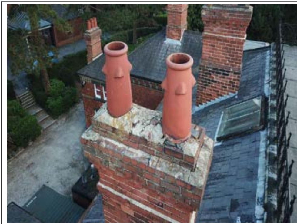
7. Cracked and friable cement flaunching.
