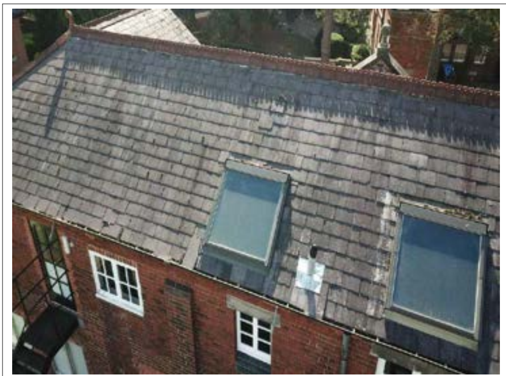
88. Slipped slates to roof covering.
