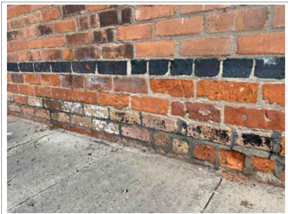
114. Retrofit chemically injected DPC.
