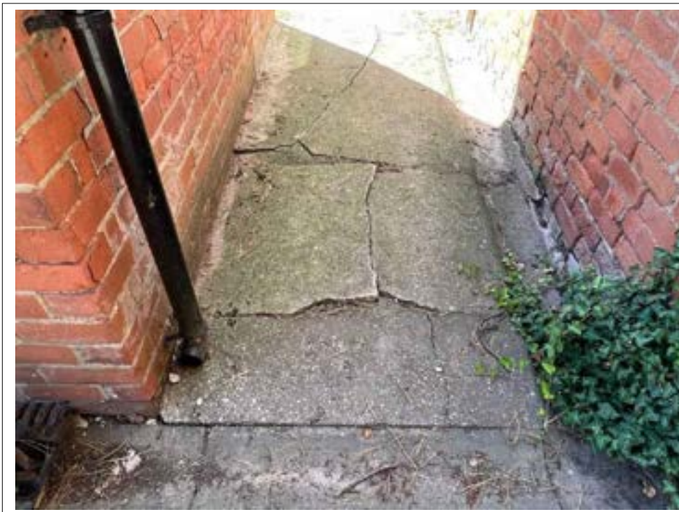
11. Concrete pathway damaged by root system.
