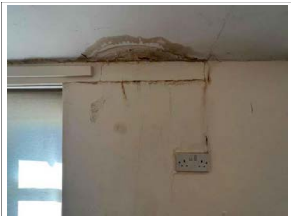
115. Water ingress to rear extension.
