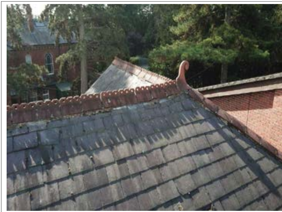
89. Cracked and friable mortar bedding to ridge tiles.
