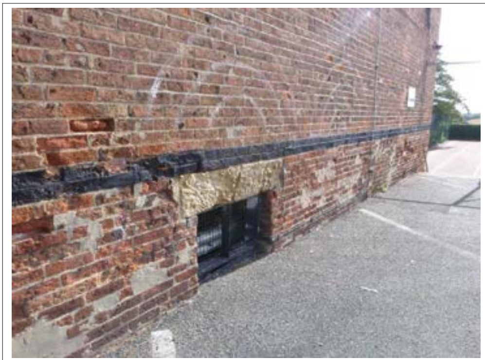
41. Frost erosion to brick masonry.
