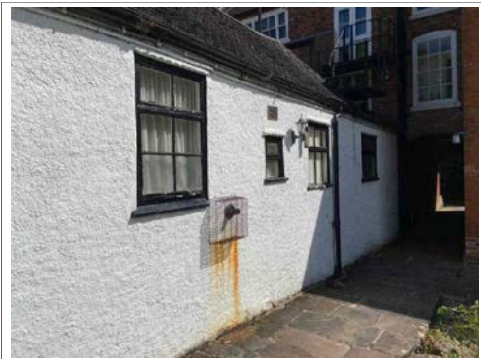
137. Corrosion to flue cage resulting in staining to elevation.
