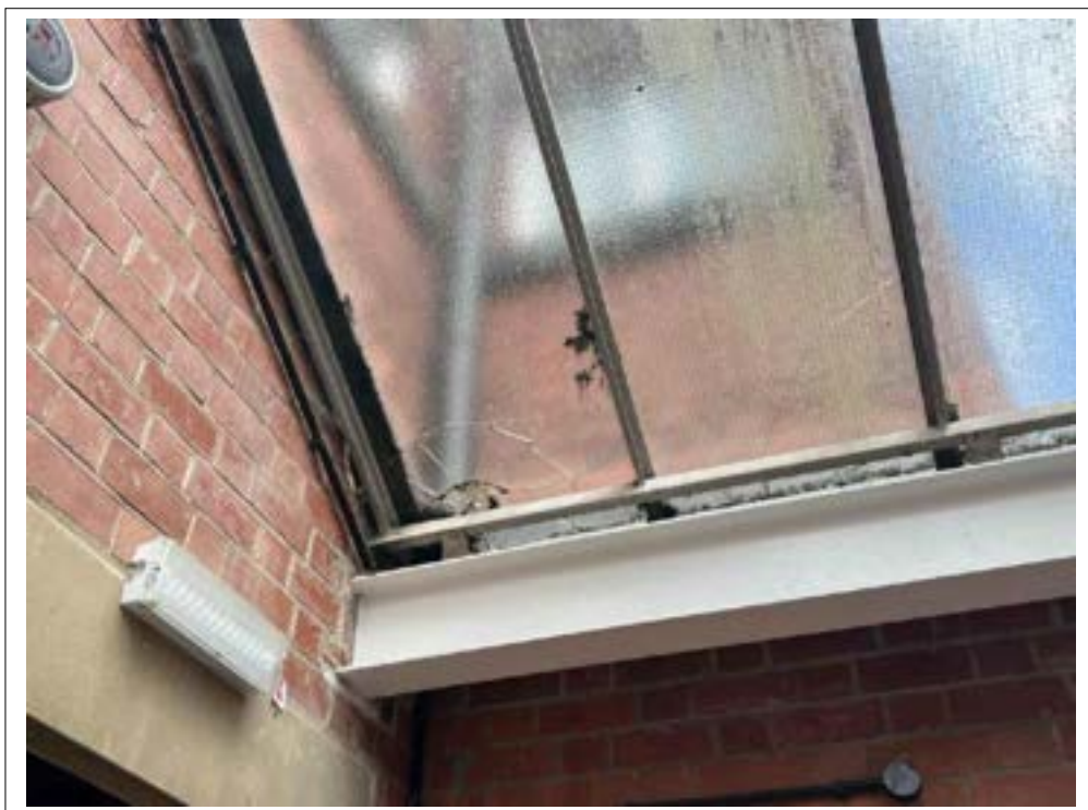
92. Cracked glazing to glazed canopy.
