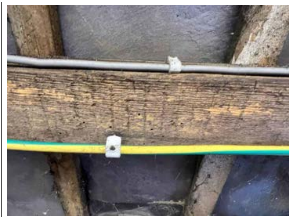
97. Flight holes noted to plant room roof structure.
