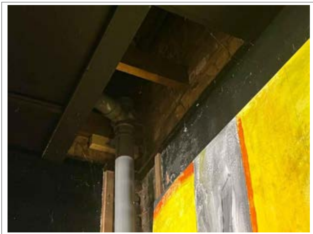
75. Ingress noted internally from internal outlet.
