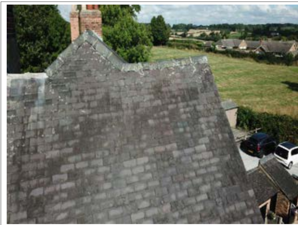
134. Soiling and lichen growth to ridge.
