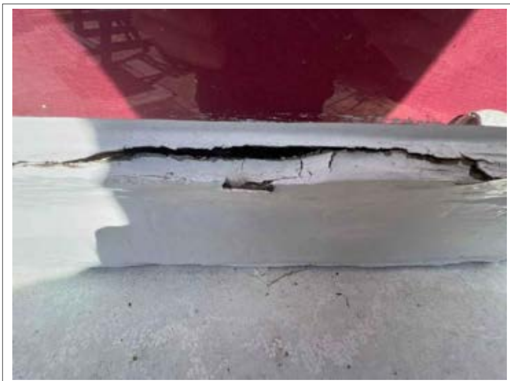
10. Wet rot to lower window cill.
