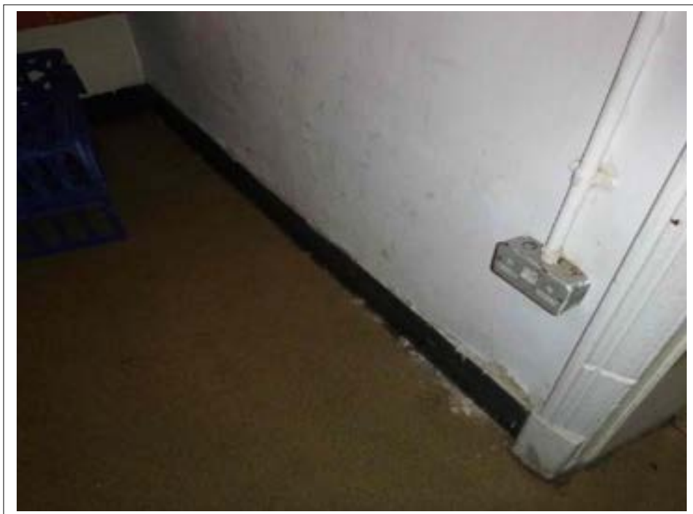
46. Isolated areas of damp ingress present at low level.
