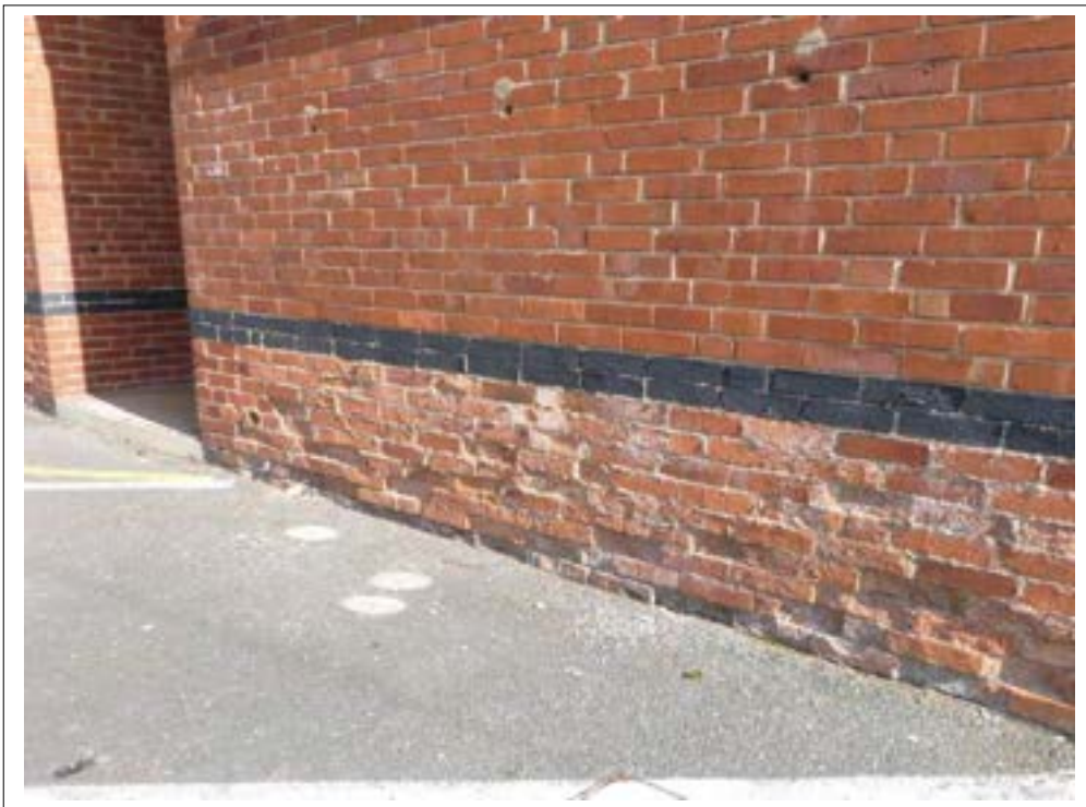
39. Frost erosion to brick masonry.
