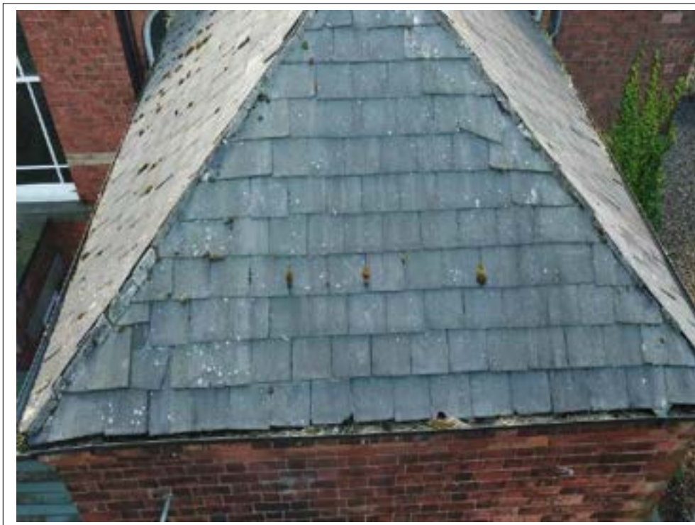
5. Missing hip tiles, slipped slates generally.
