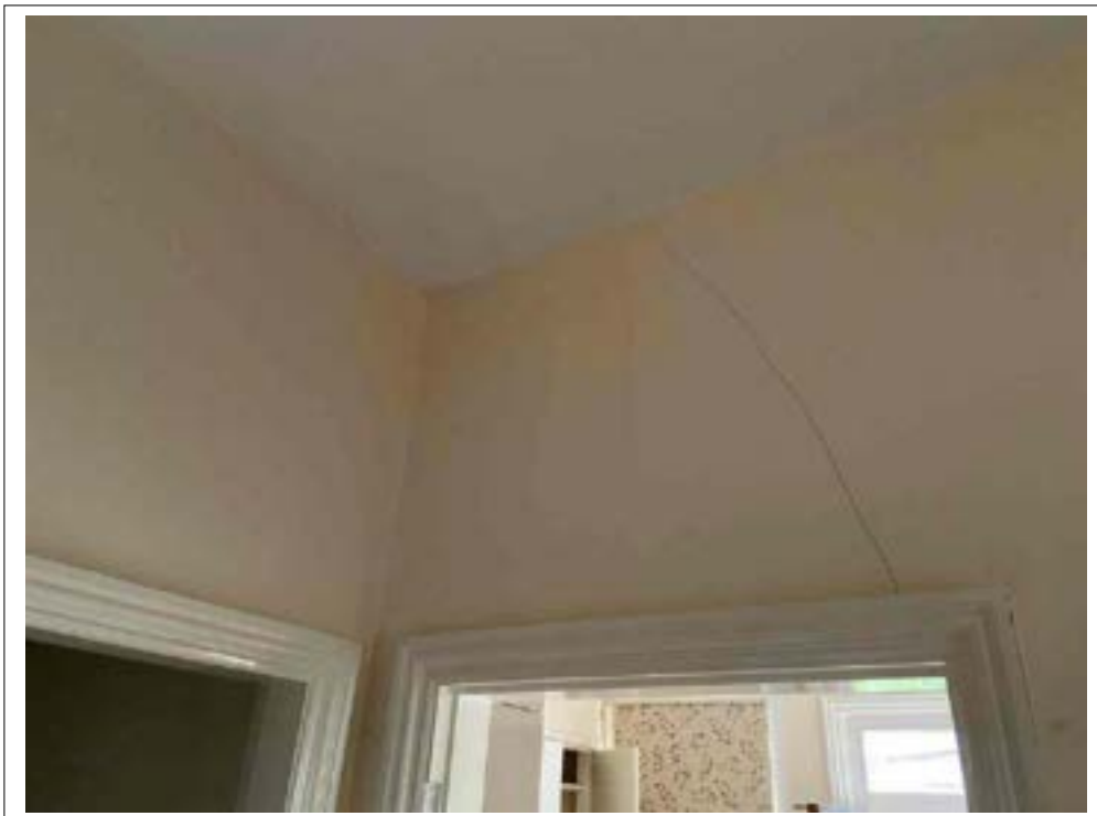
126. Crack noted internally.
