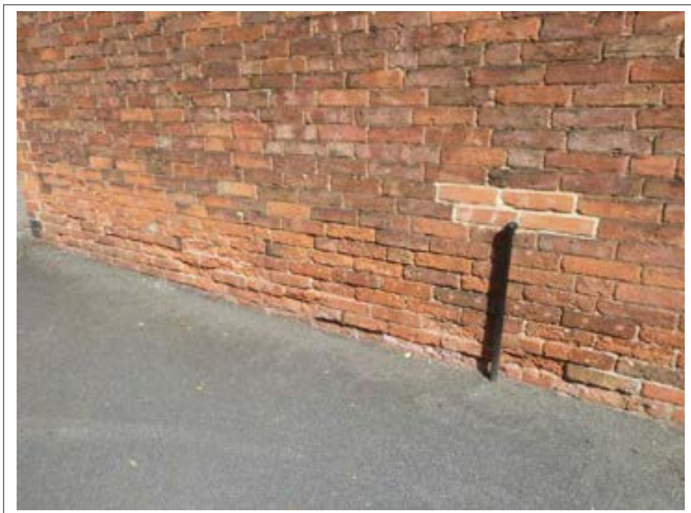
159. Frost erosion to brickwork.
