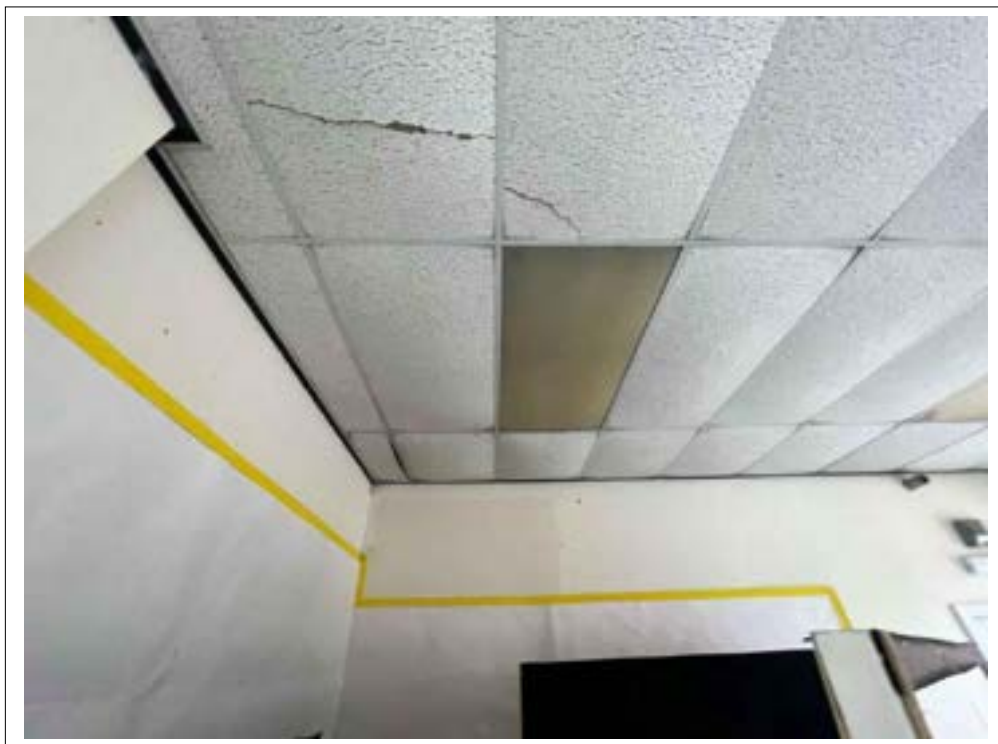
93. Cracked ceiling tiles with undulations noted generally.
