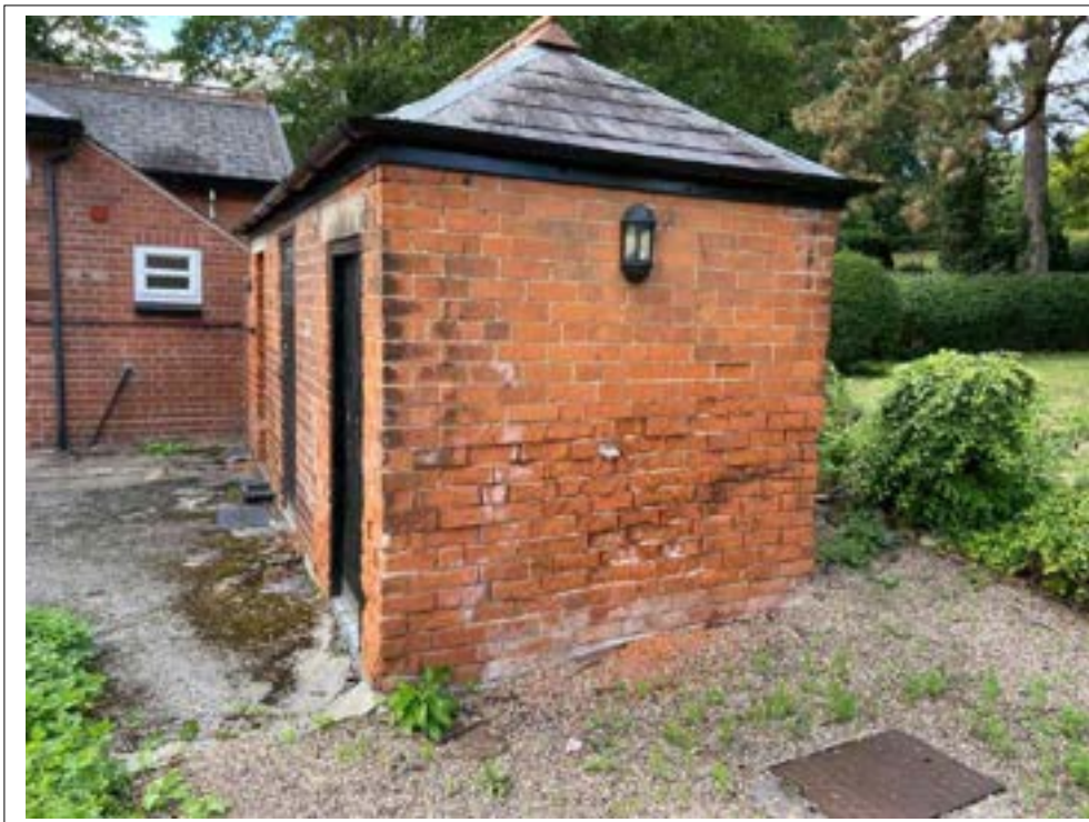
124. Frost erosion to brickwork to outhouse.
