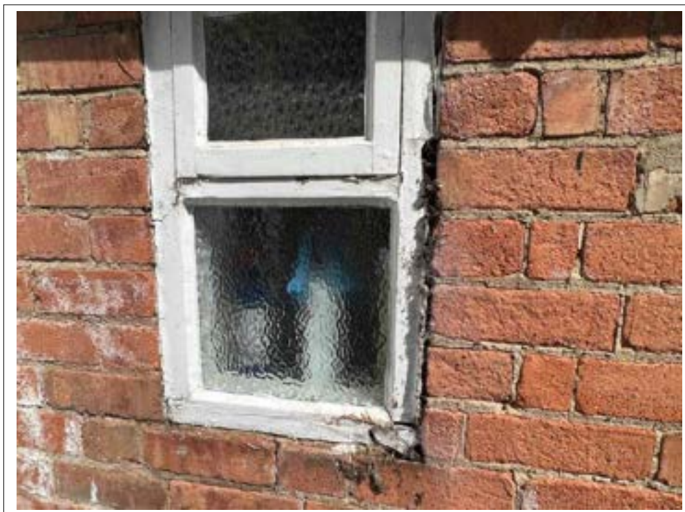
112. Wet rot to timber window.
