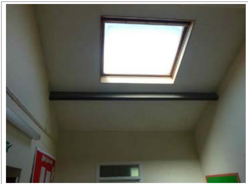
62. Localised water staining around rooflight.
