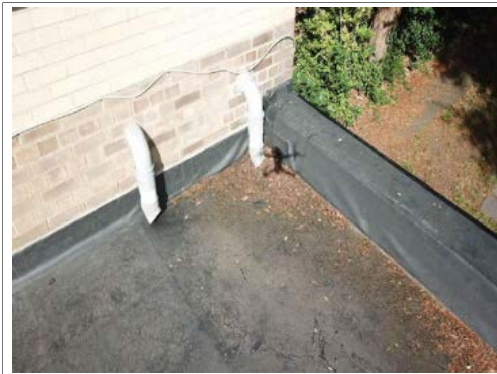
67. Single ply membrane lifting.
