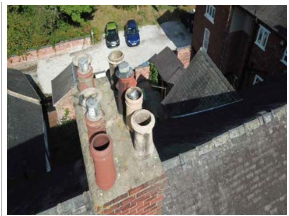
131. Cracking to cement flaunching.
