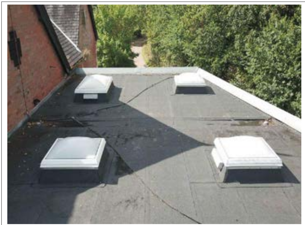
168. Felt flat roof covering.
