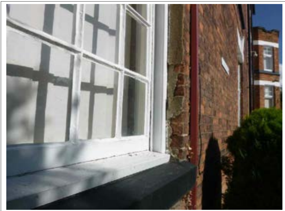
27. Spalling to window surround.
