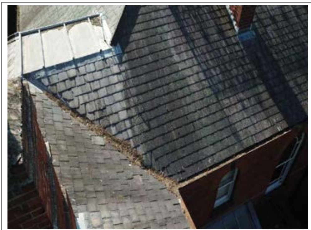
4. Vegetation build up to rainwater goods.
