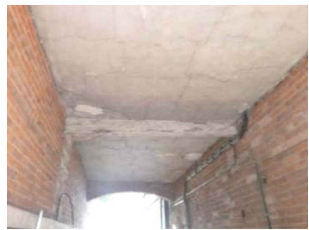
138. Cracking noted to alleyway soffit.
