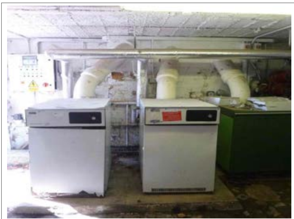
63. Gas boilers to basement area.
