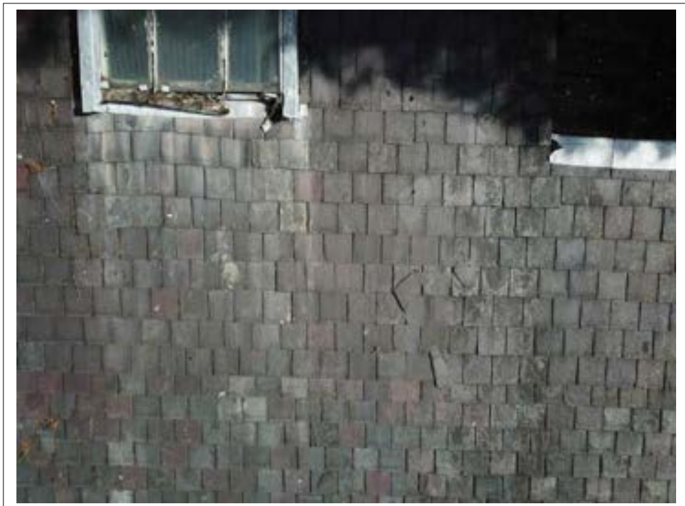
108. Slipped slates to South extension, decayed rooflight.
