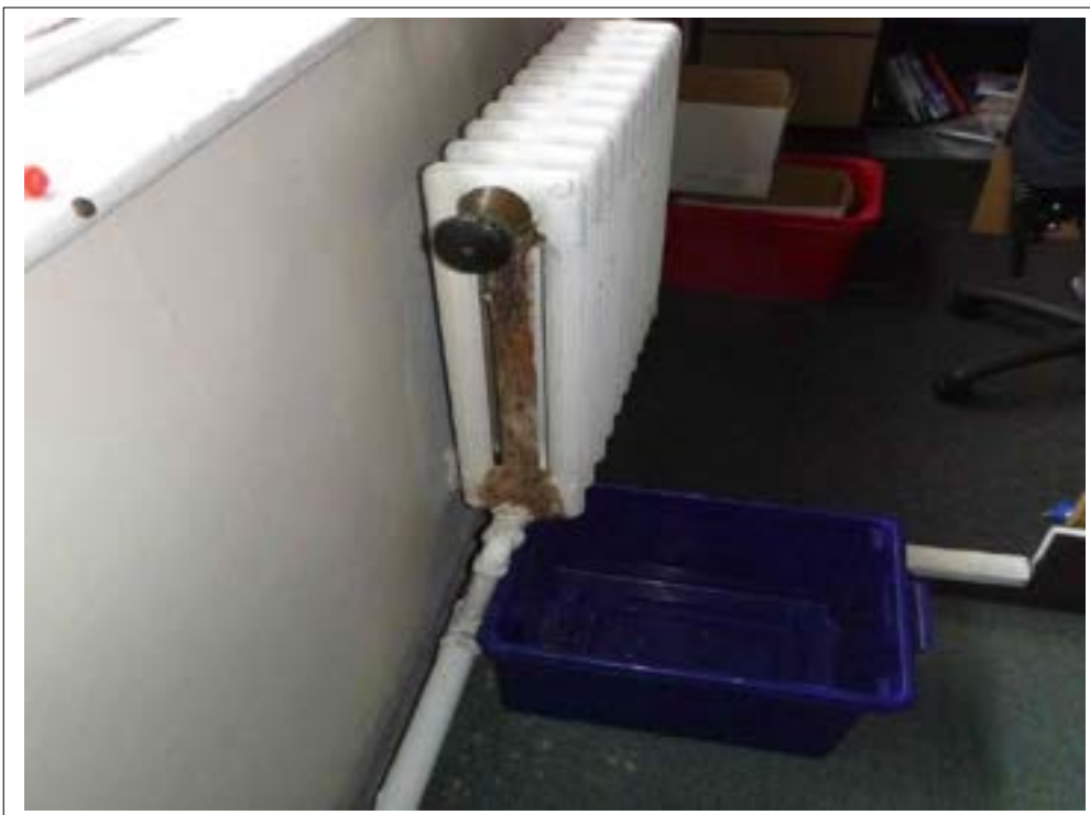
58. Defective valve to radiator.
