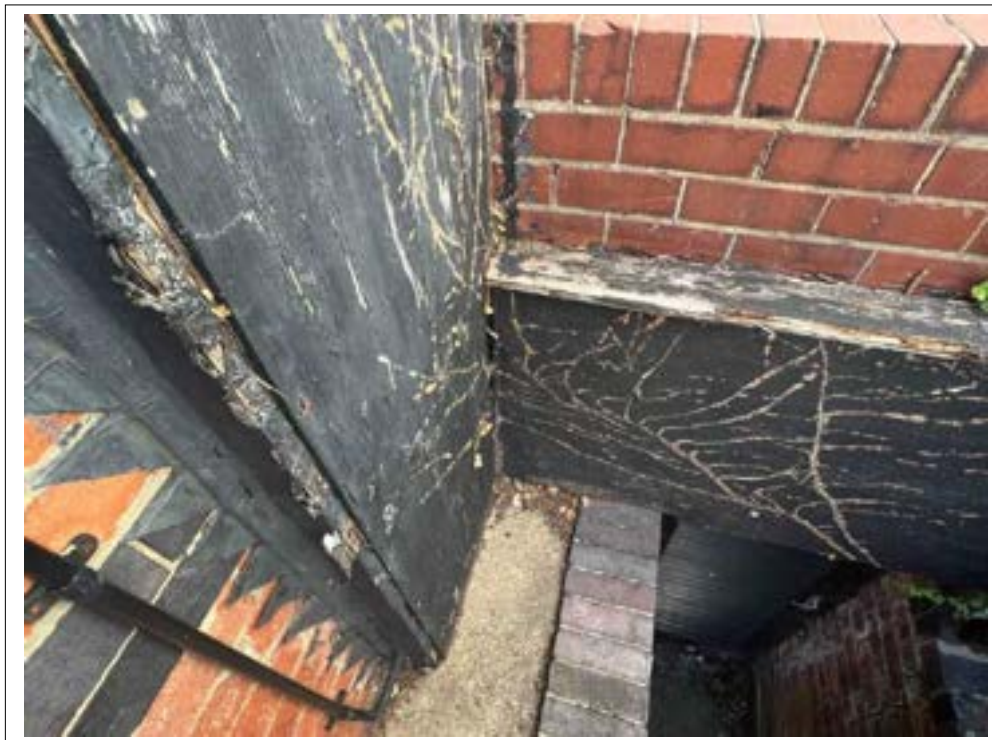
71. Wet rot to timber service housing.
