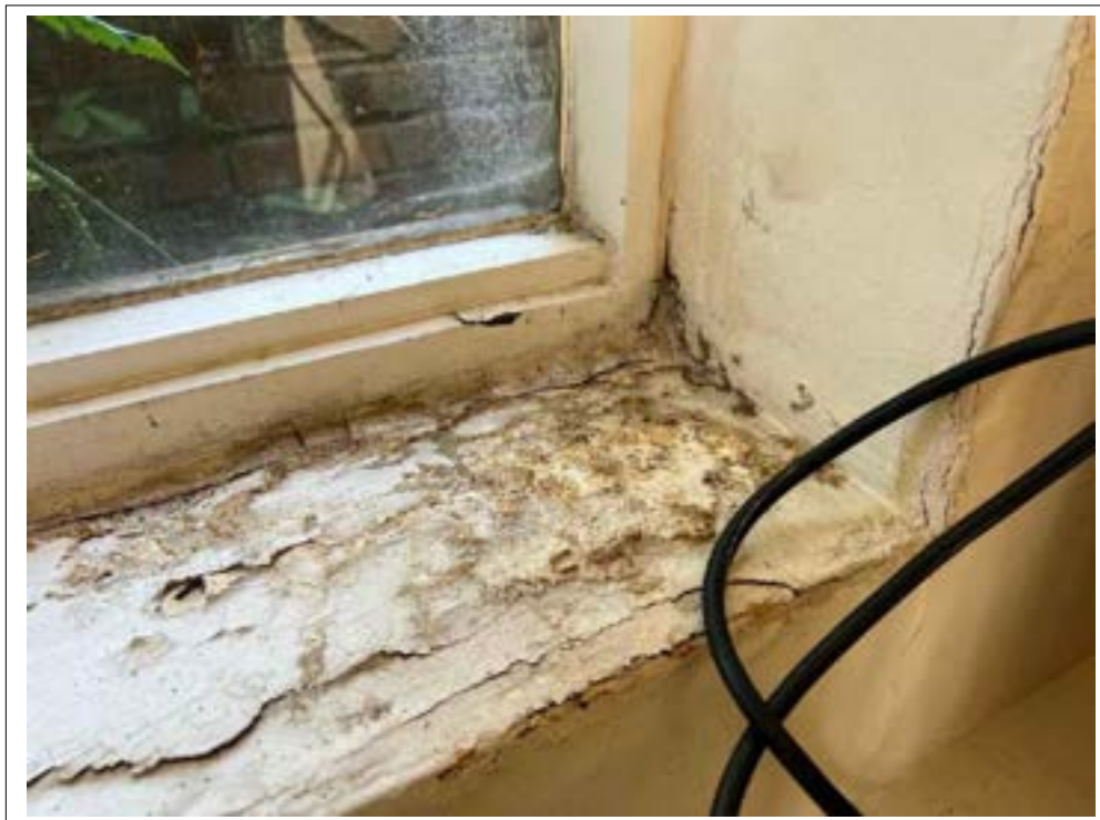
73. Damp ingress to West elevation window reveal.
