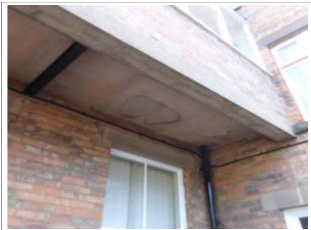
33. Spalling to soffit.
