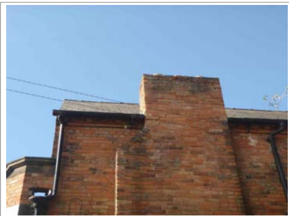
30. Cracking to chimney breast.
