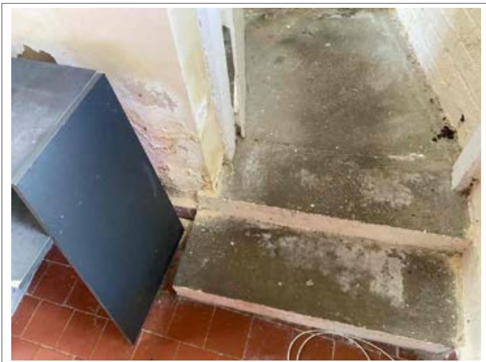
149. Isolated damp ingress to west extension laundry room.
