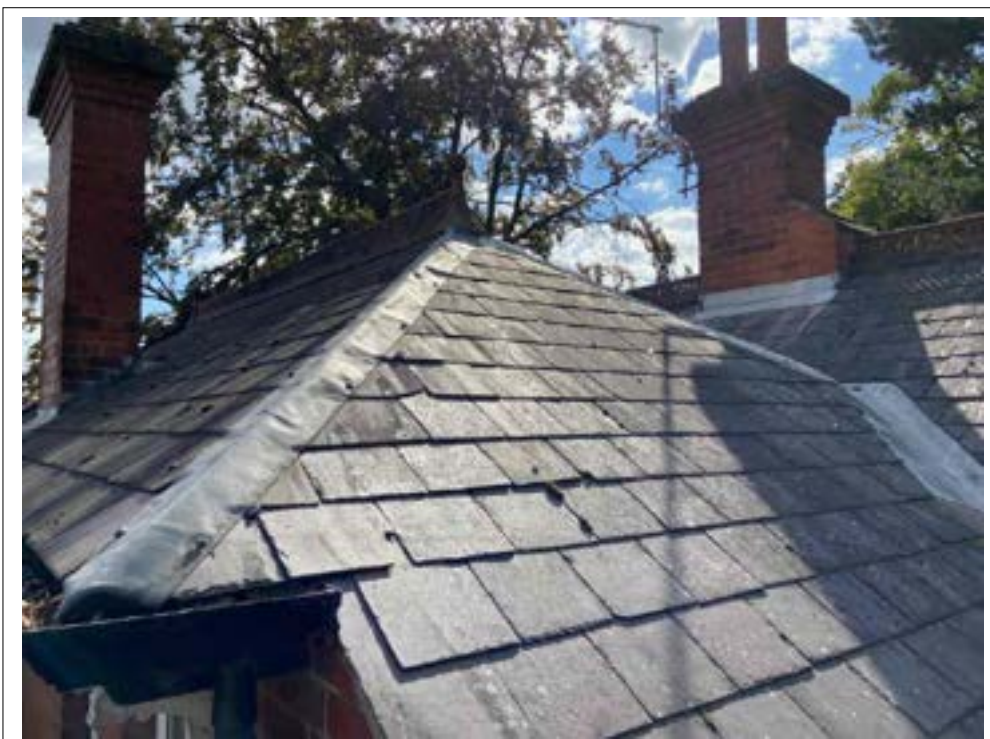
121. Mechanically fixed hip flashing.
