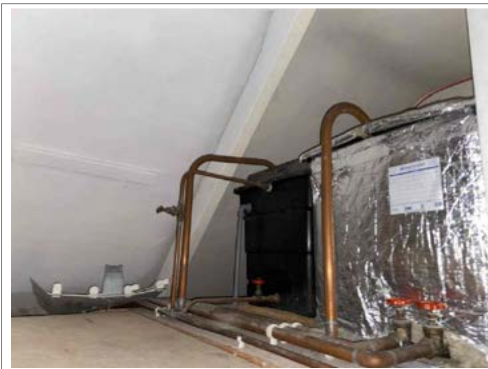
148. Water storage tank to roof void plant room.
