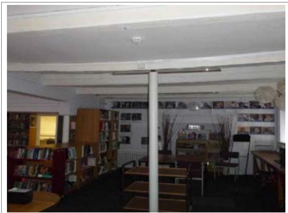
47. West extension, south wing, interim steel support to timber floor.
