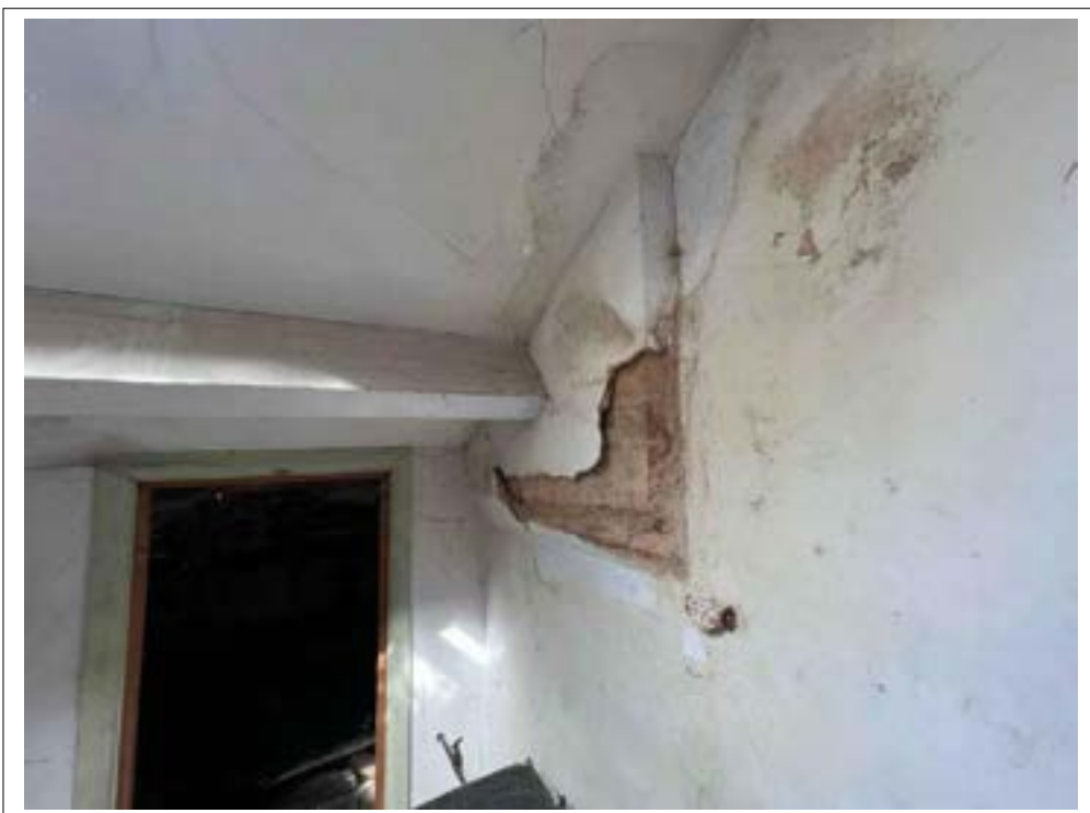
14. Damp ingress and blown plaster.
