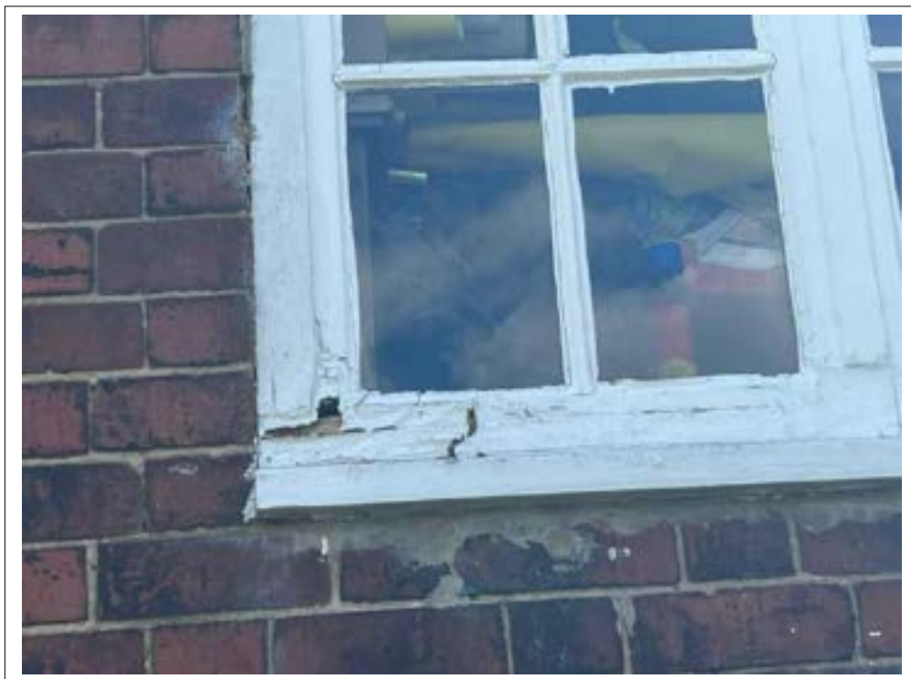
91. Wet rot to lower cills and frame.
