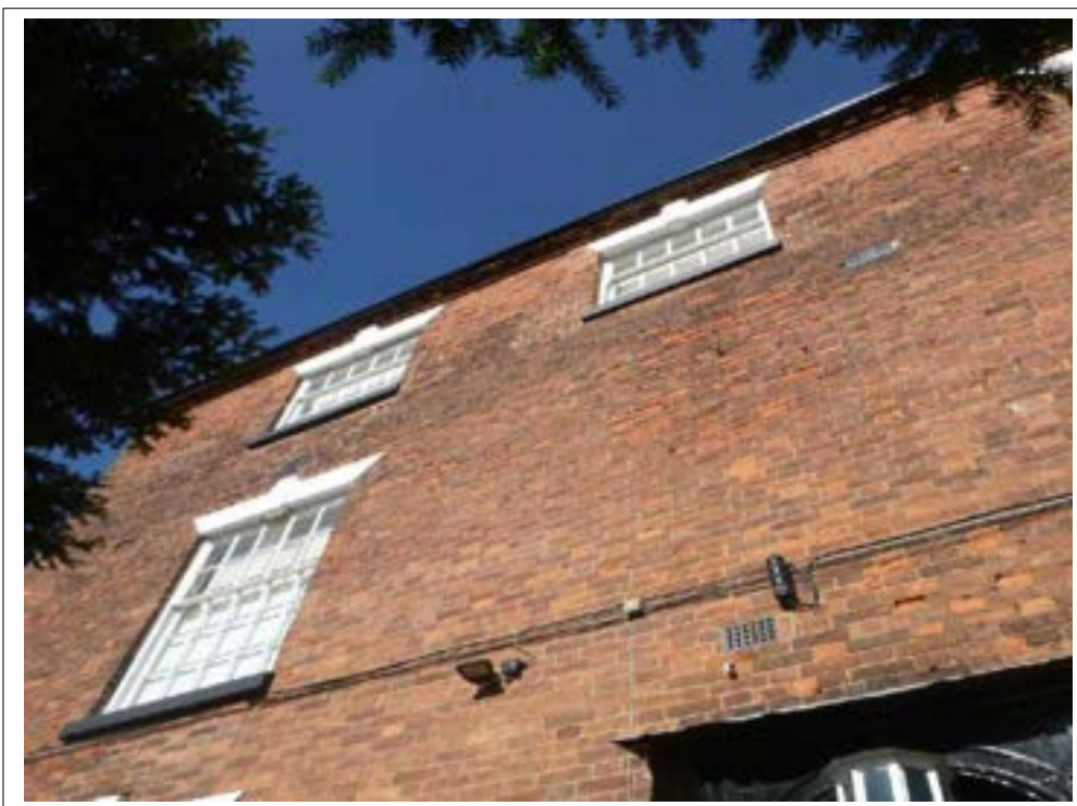
26. East elevation, weathered brickwork.
