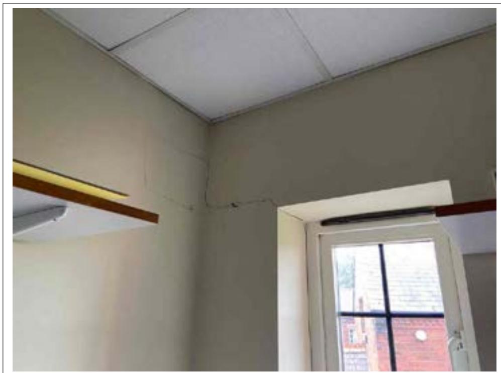
82. Settlement cracking to south east corner.
