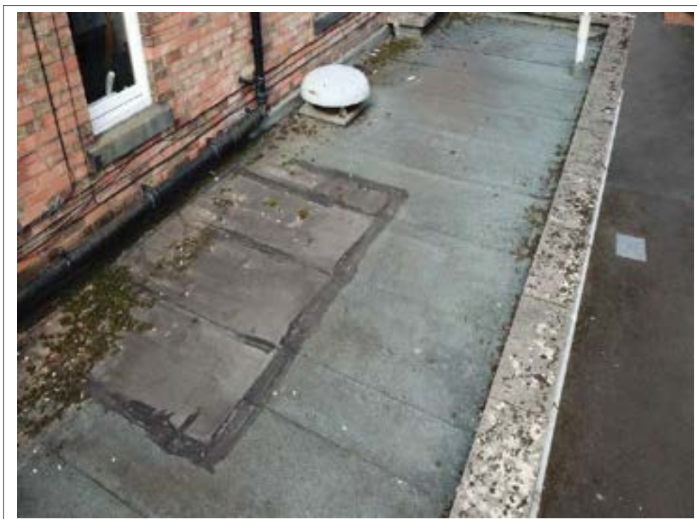
24. Evidence of patch repairs to flat roof.
