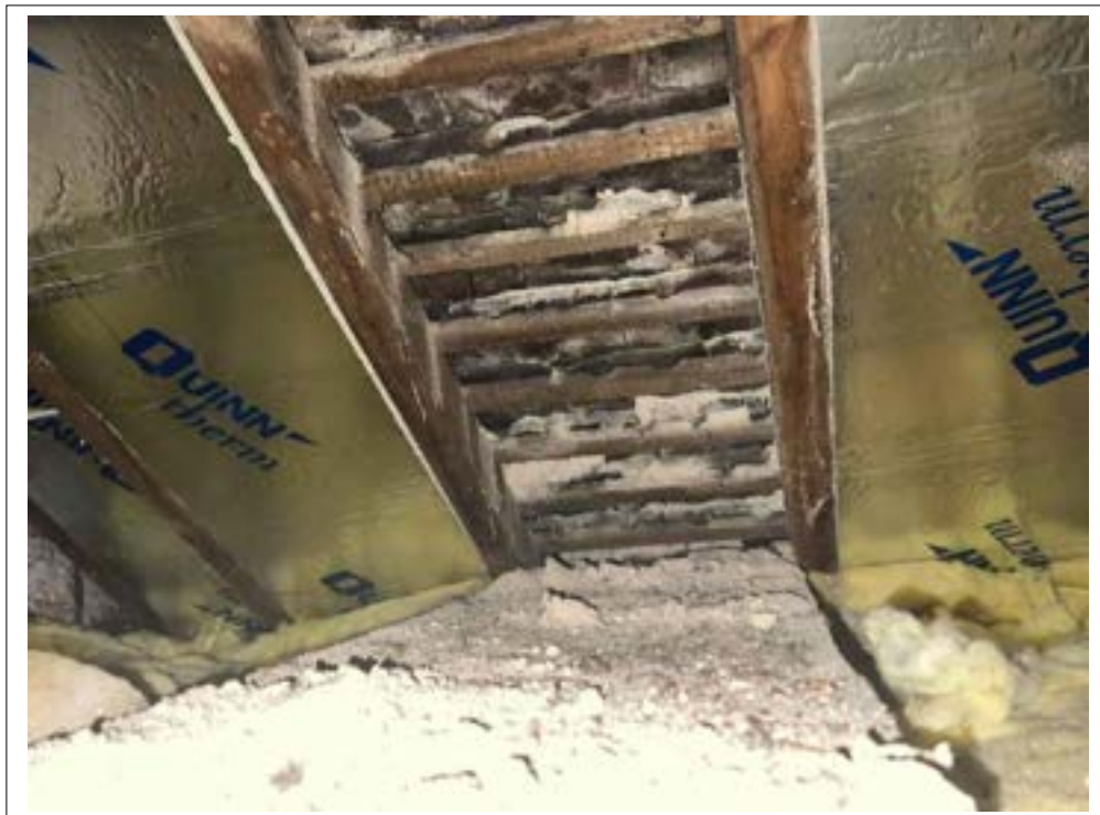
183. Roof void with rigid board insulation present.
