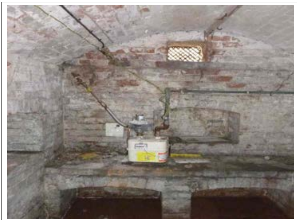
161. Basement and incoming gas supply.
