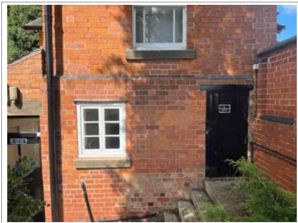
110. Movement noted to low level brickwork.
