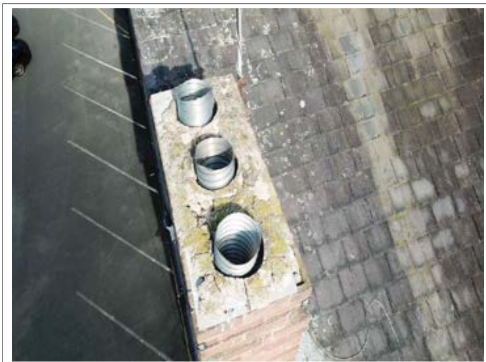
22. Cracked flaunching to chimney.
