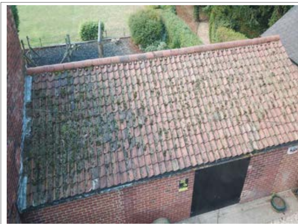
6. Foliage build up to roof covering.
