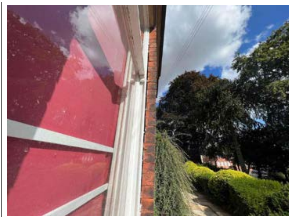
9. Bowing noted to brick pier to East elevation.
