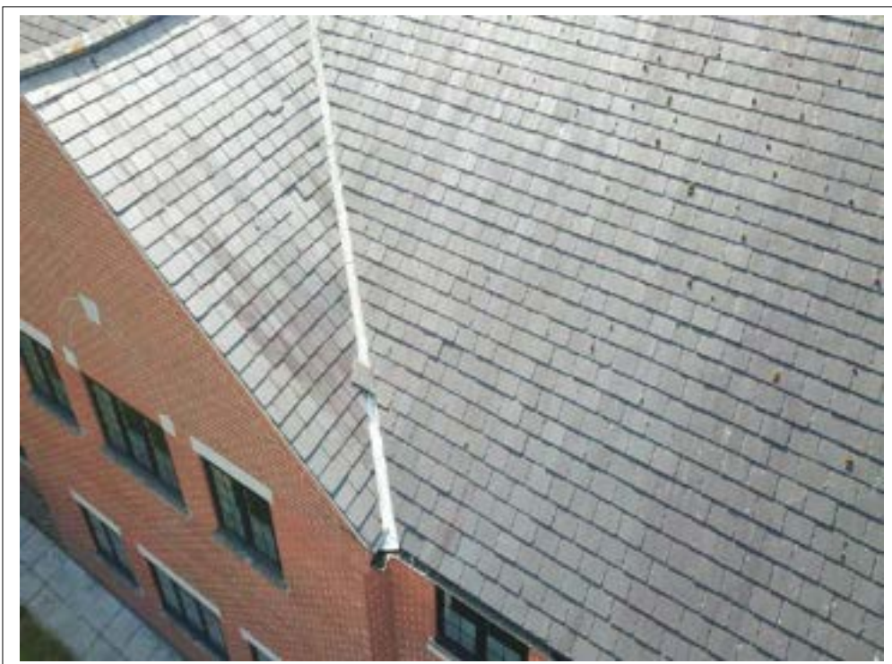
77. Slipped slate to valley gutter.
