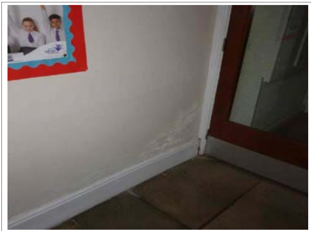
44. Isolated areas of damp ingress present at low level.
