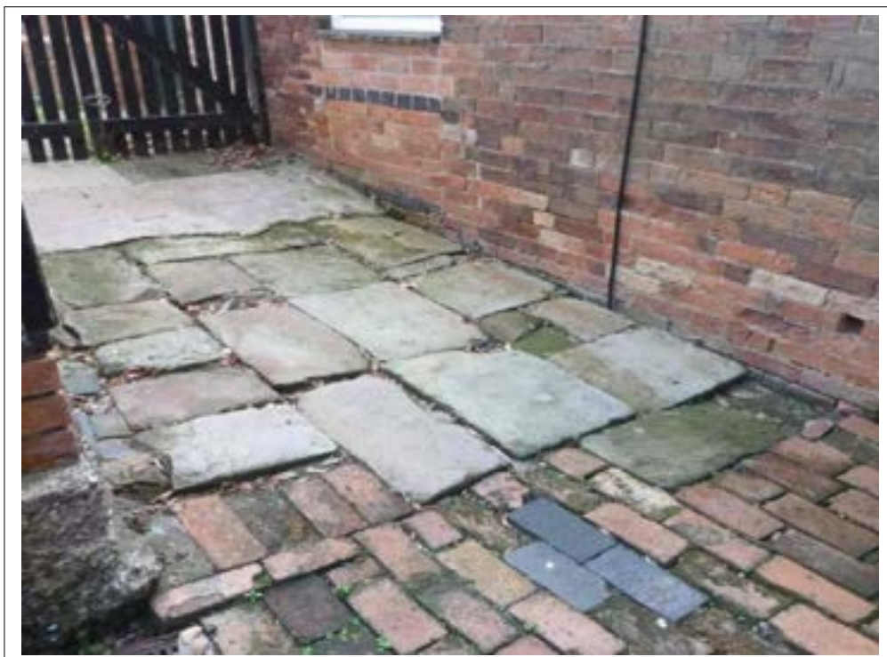
160. Undulating paving surface to rear pathway
