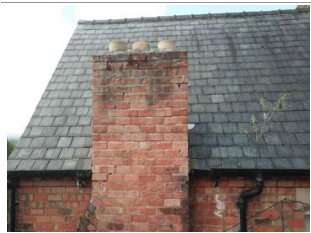
25. Cracking to chimney breast.
